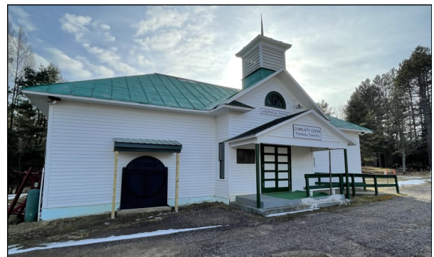
Lugerville School with display on left. Photo by John L. Berg
