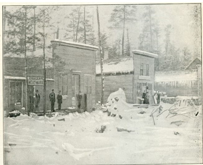
Lake Street during the first winter in Phillips, Town of Worcester, Chippewa County, Wisconsin, 1876–1877. From A Glimpse at the Early History of the State of Wisconsin Relating to Price County. , ca. 1906
